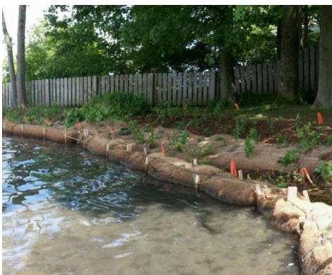
Fig. 9. Coir (coconut fiber) logs are a type of bioengineered erosion control.
