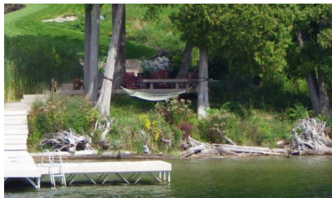
Fig. 10. Intentionally placed stumps and brush bundles are also used for bioengineered erosion control.
