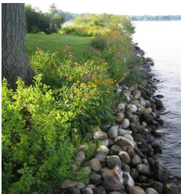
Fig. 5. Narrow, unmowed vegetation belt, above sloped artificial erosion control
