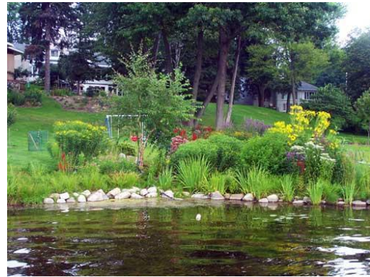
Fig. 8. Sloped artificial erosion control includes rock and riprap, even in minor amounts.
