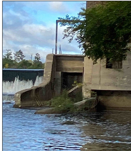
Stoplog Auxiliary Spillway
