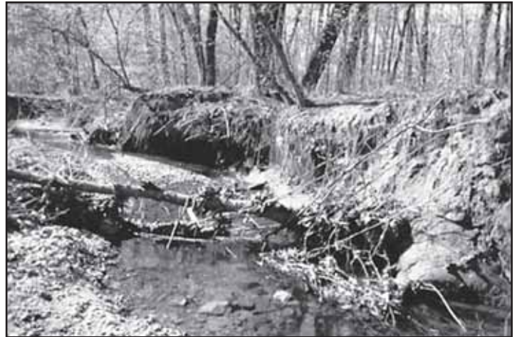
Millers Creek flows through Ann Arbor. The severely eroded streambanks and channel result from development in the creekshed. Photo: HRWC
