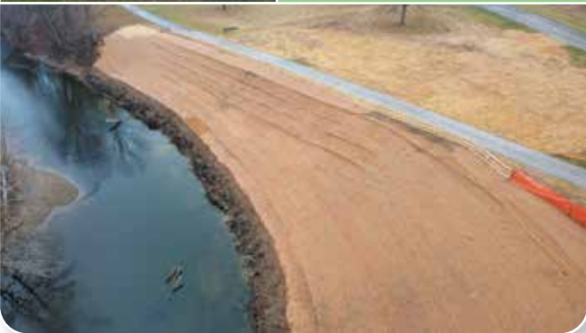
Bank of Big Bend before (showing bank encroachment towards the road) and an aerial view after the restoration. Note toe wood at the water line and a flat planting bench just above. credit: Metroparks
