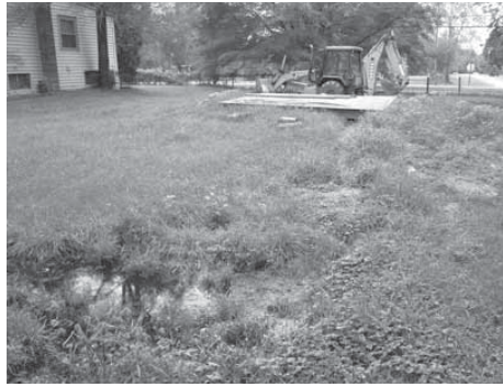
Indications of a septic failure in the summer include lush vegetation due to the excessive nutrient release and standing water (left). In the winter, failing septic systems can be identified by melted snow caused by warm septage leaking up through the ground (right). photo: Washtenaw County
