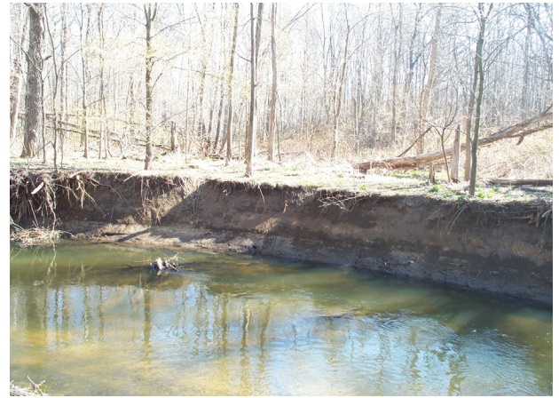
Before. Bare, vertical banks at this site were the result of dredging and upstream changes to hydrology in Mill Creek.
