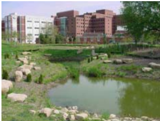
CH2M Hill designed this wetland stormwater detention basin complex for the University of Michigan's North Campus. —photo: CH2M Hill
