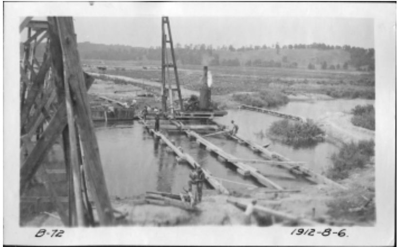
The beginnings of Barton Dam, 1912. —Gardner Stewart Williams Papers, Bentley Historical Library, University of Michigan
