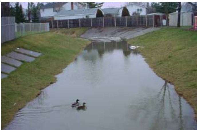
Cass Drain, a tributary in the Lower Huron River Watershed, typifies a problem found in most drains: lack of riparian vegetation. —photo: R. Schrameck
