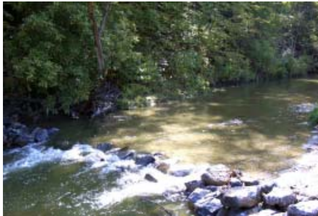
Installing boulder drops, like those shown here, are one recommendation of the Millers Creek Improvement Plan. —photo: Frederick-Winchester Service Authority
