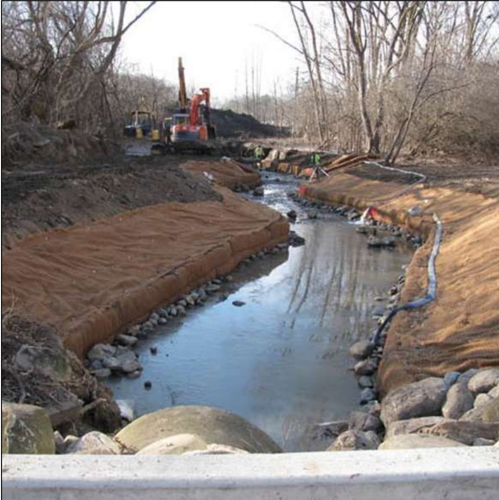
Stream reshaping at County Farm Park
